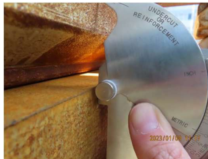
鋼柱對接板位差查驗
