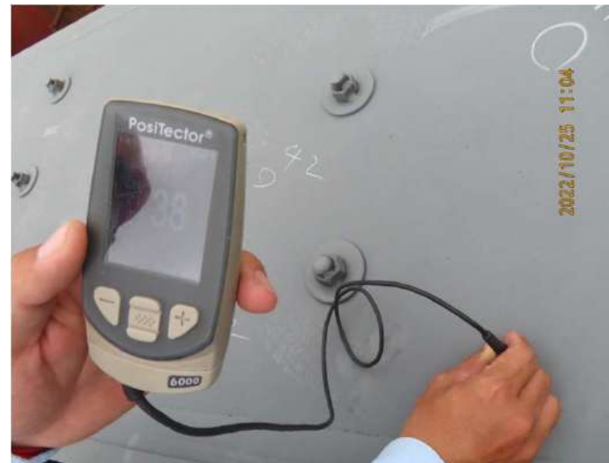
鋼梁乾膜厚度查驗
