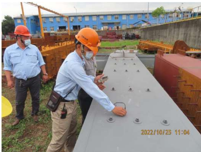
鋼梁乾膜厚度查驗
