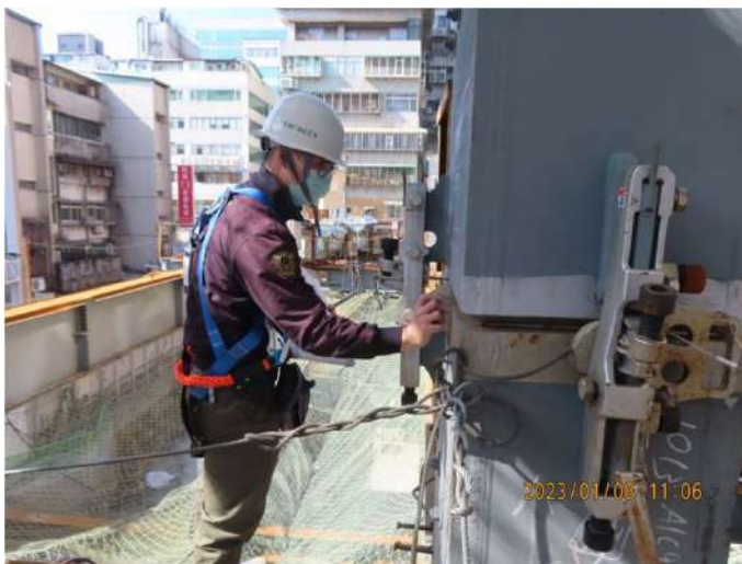
鋼柱對接板位差查驗
