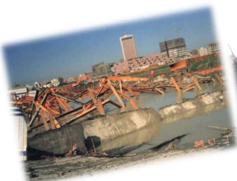
Heave due to push-in of retaining wall
