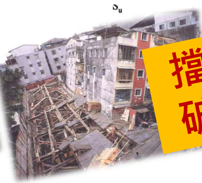
Heave due to Plastic Flow of Soft Clay
