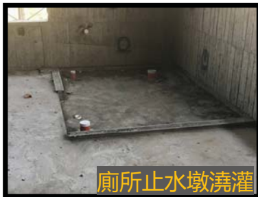
廁所止水墩澆灌
