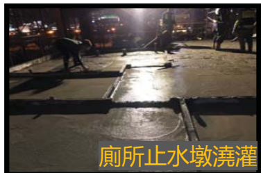
廁所止水墩澆灌
