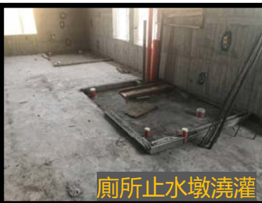
廁所止水墩澆灌
